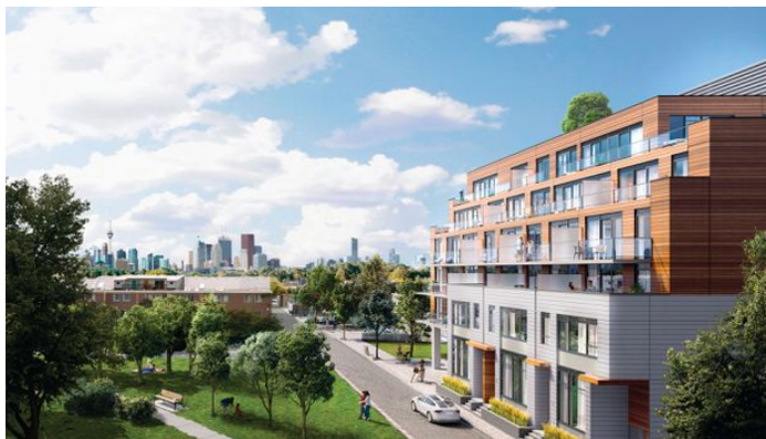
A rendering of Fieldgate Urban's The Poet development at 1285 Queen Street East in Toronto.
