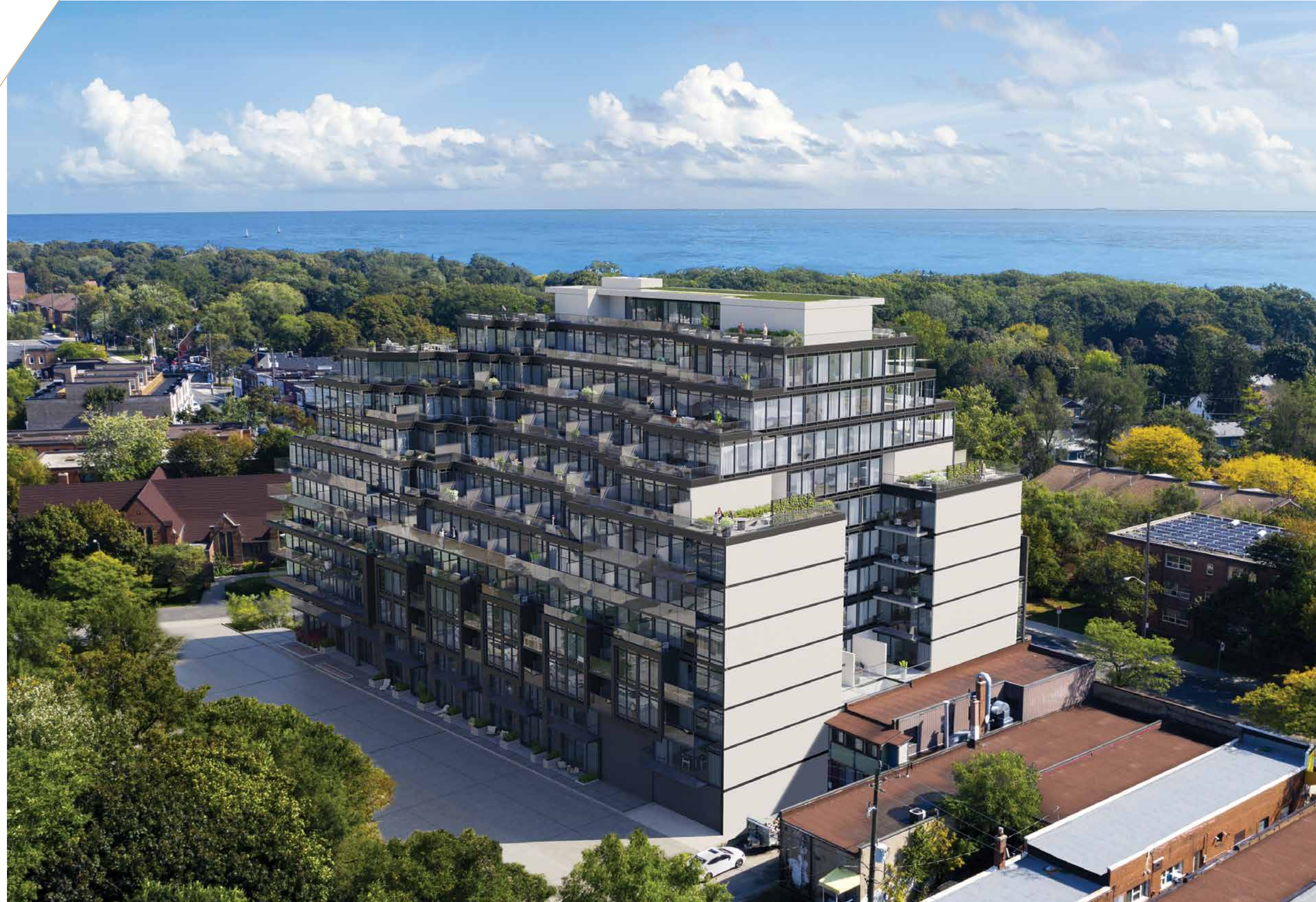
The sophisticated terraced design figures prominently on the north façade.
