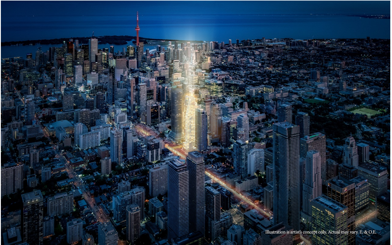
Looking southwest to 8 Wellesley | Residences at Yonge, image courtesy CentreCourt/Bazis
