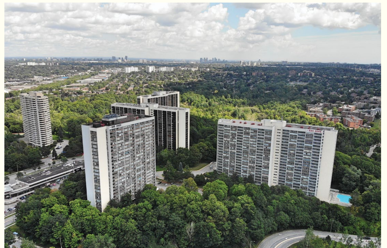
WYNFORD HEIGHTS CRESCENT, TORONTO
