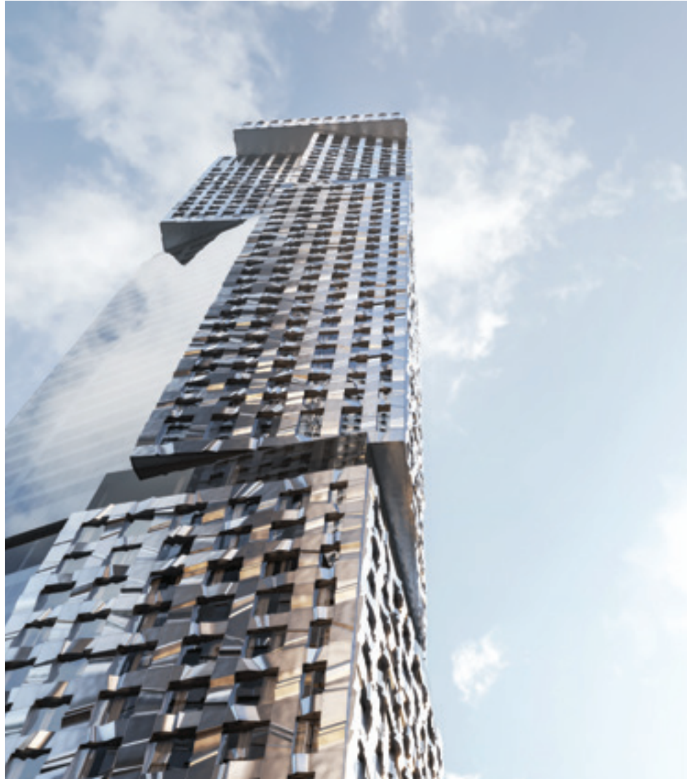
East Tower Façade
