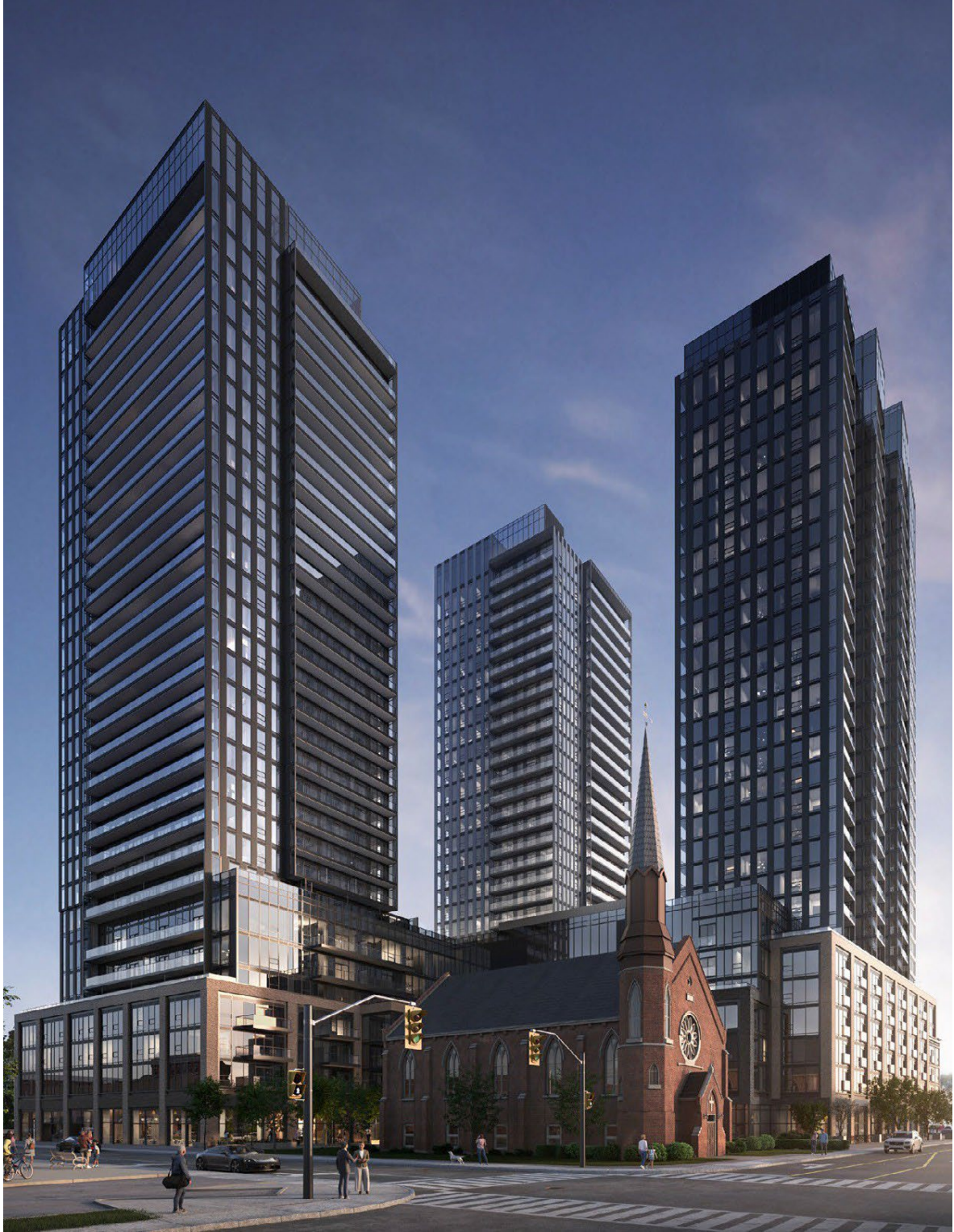
THE DESIGN DISTRICT Hamilton 334 Suites (Tower C)
