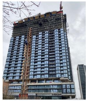
Windows installed up to the 20<sup>th</sup> floor, balcony railings up to the 14<sup>th</sup> floor, corridor drywall is up to the 18<sup>th</sup> floor, suite framing up to the 16<sup>th</sup> floor and suite drywall up to the 12<sup>th</sup> floor
