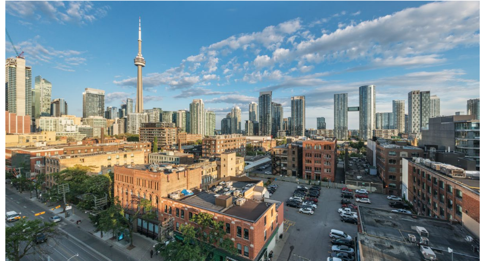
ABOVE: Current storefronts and heritage buildings on site
