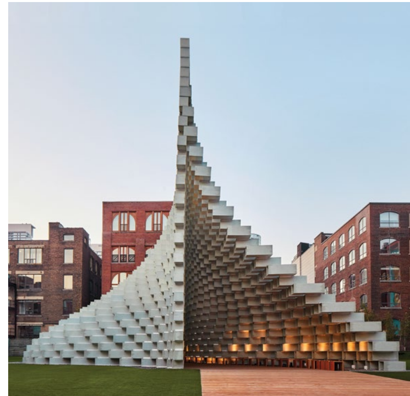
The 2016 Serpentine Pavilion Bjarke Ingels
