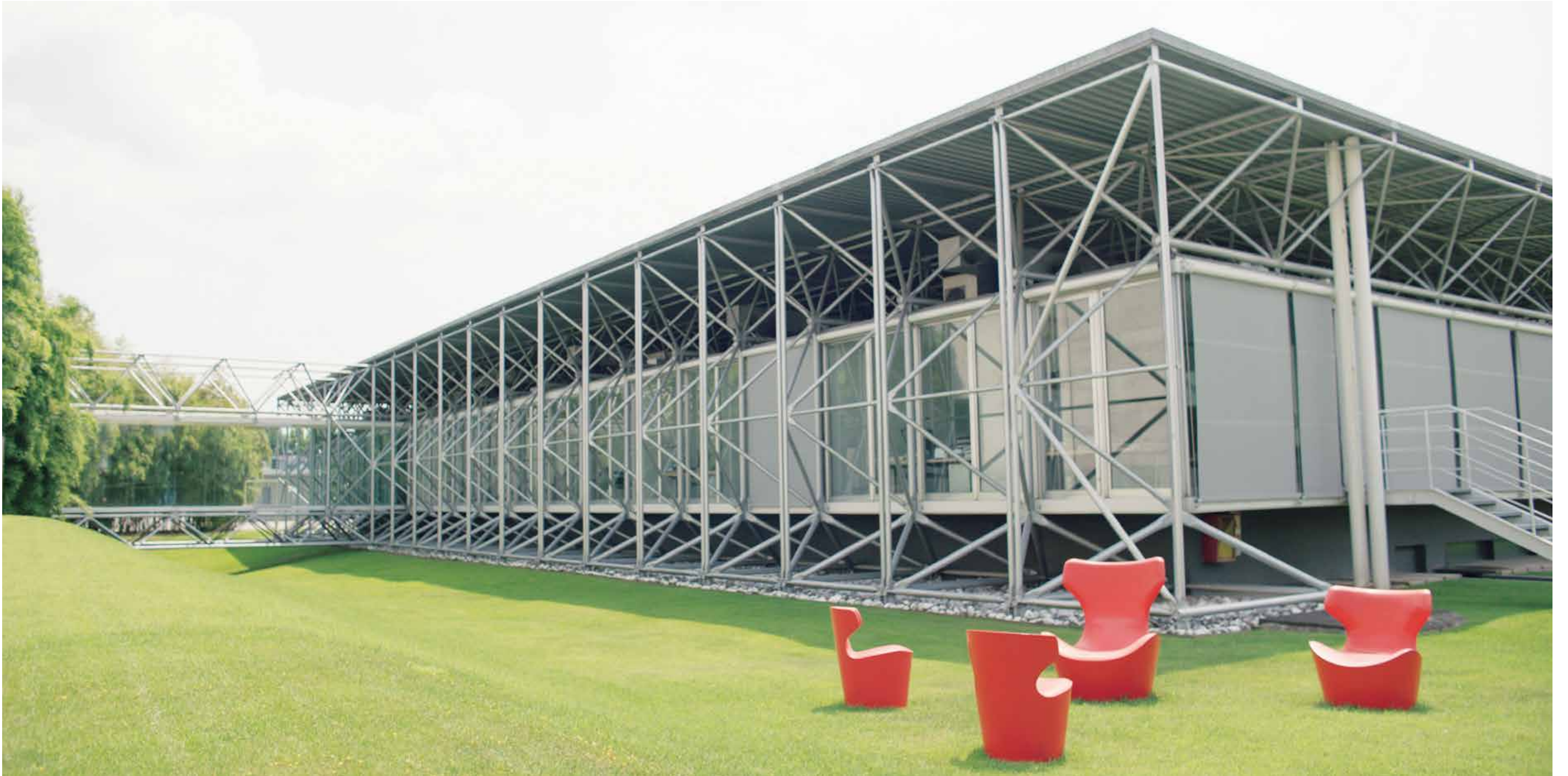
ABOVE: BBB Italia's headquarters in Novedrate, Italy.
