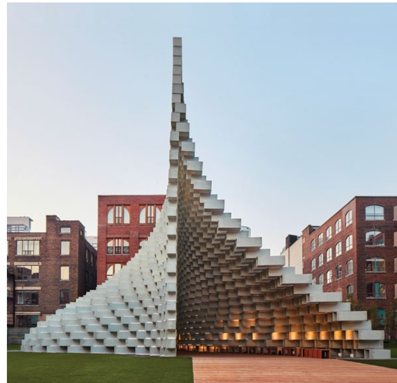
The 2016 Serpentine Pavilion Bjarke Ingels
