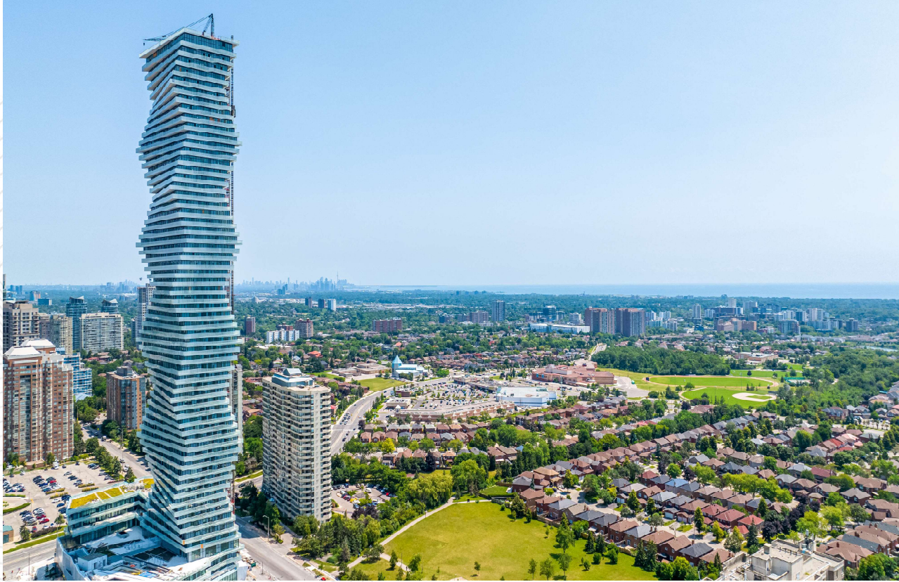
35 th Floor – Southeast View
