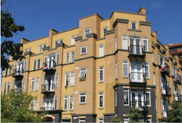
Apartment buildings can provide visual interest and articulation by using such features as balconies, corner treatments and a step-back on the top floor.
