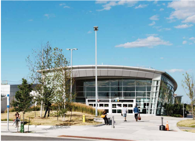
Downsview Park Subway Station
